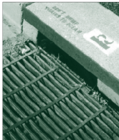
Storm drains, like the one shown here, flow directly to the ocean. Goleta West Sanitary District's sewers flow to the wastewater treatment plant.
